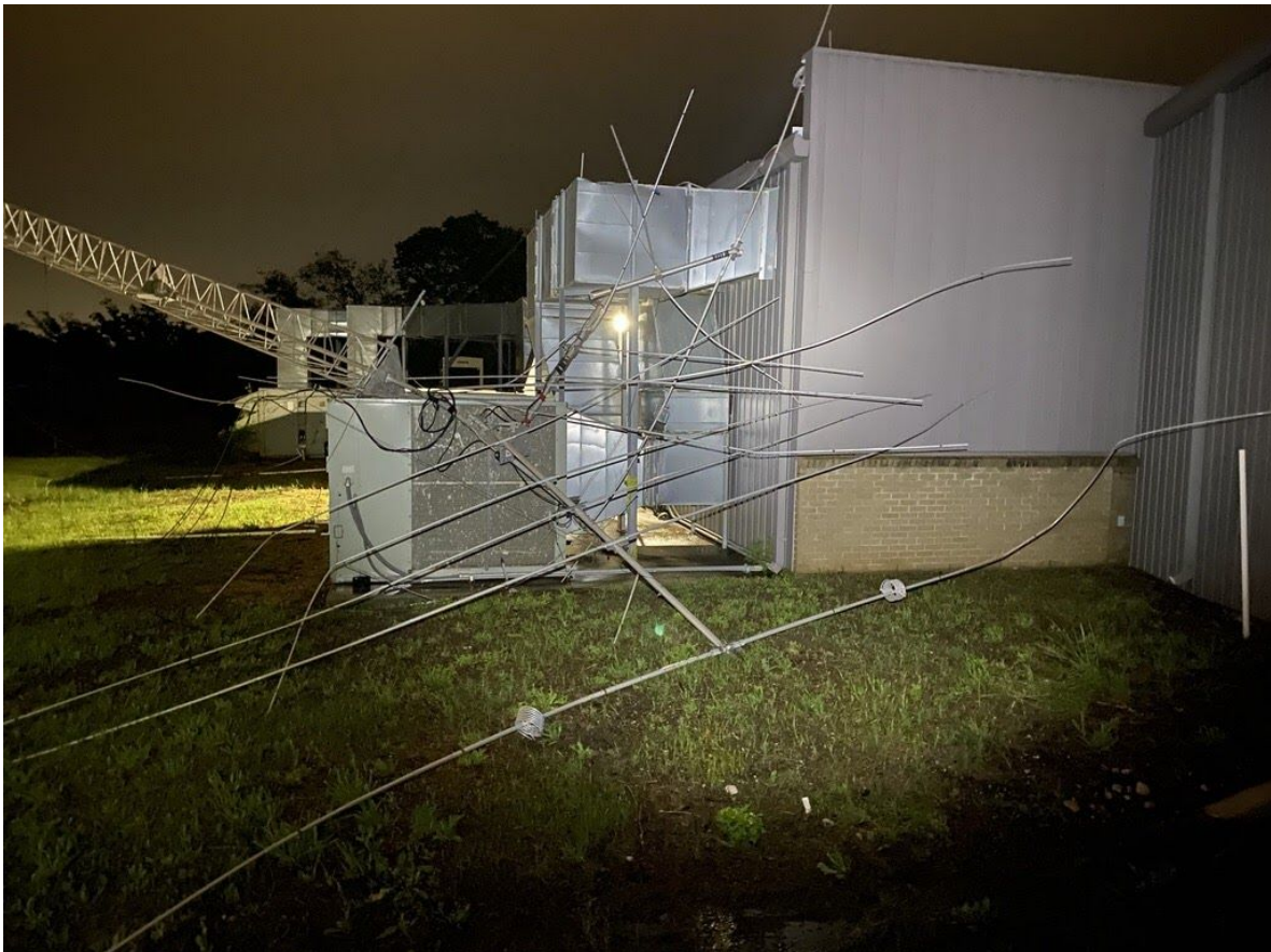
A wider shot of the damage to the Force 12
